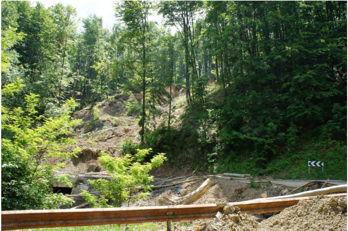
Figure 4.9 - Debris flow seen in the valley above the Antimony Mine Waste Tailings Dam where damage to the road and road infrastructure was observed.
