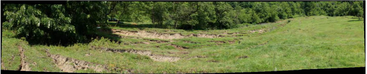
Figure 4.1 - Scarp features seen in the middle of the landslide mass at Mali Zvornik showing typical features for multiple rotational slides.
