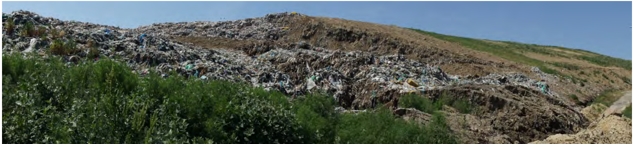
Figure 4.11 - Scarp features seen in the middle of the landslide mass at the Belgrade Municipal Waste site showing typical features for multiple rotational slide.
