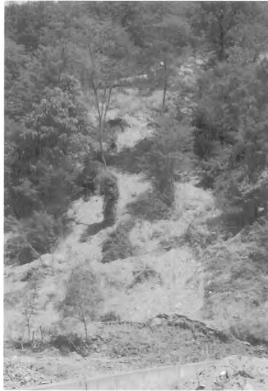
Debris flow in the weathered shales
