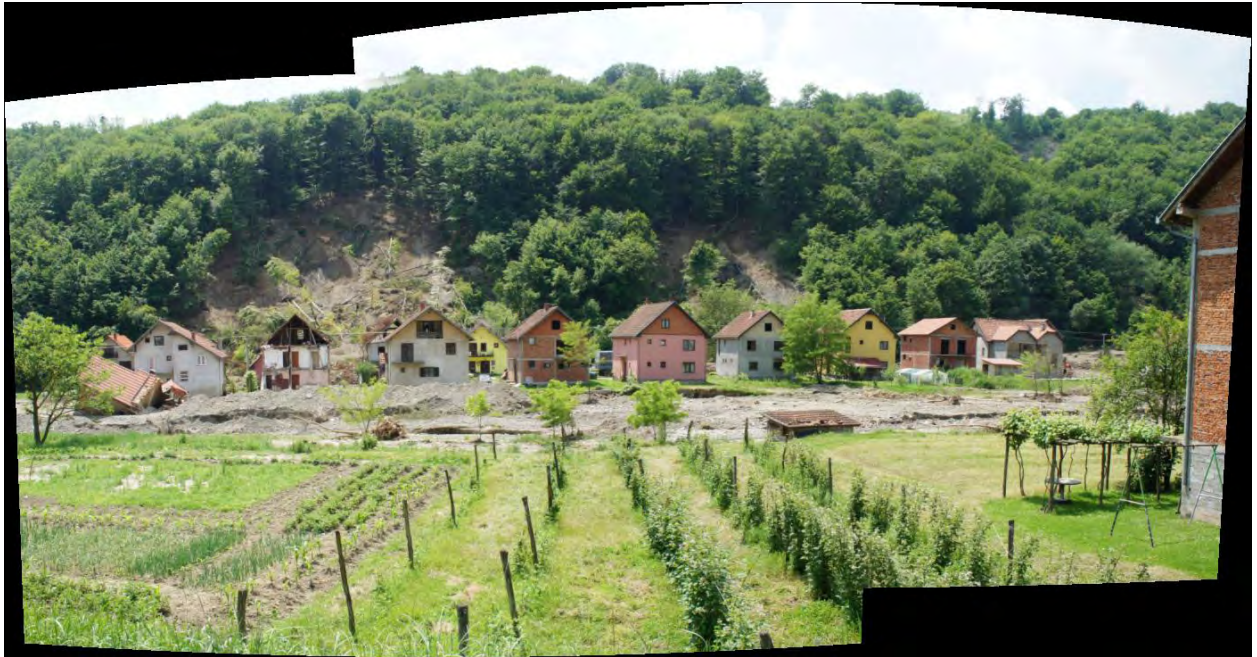
Figure 4.7 - Debris slides seen in the Cadjavica valley that have damaged houses.
